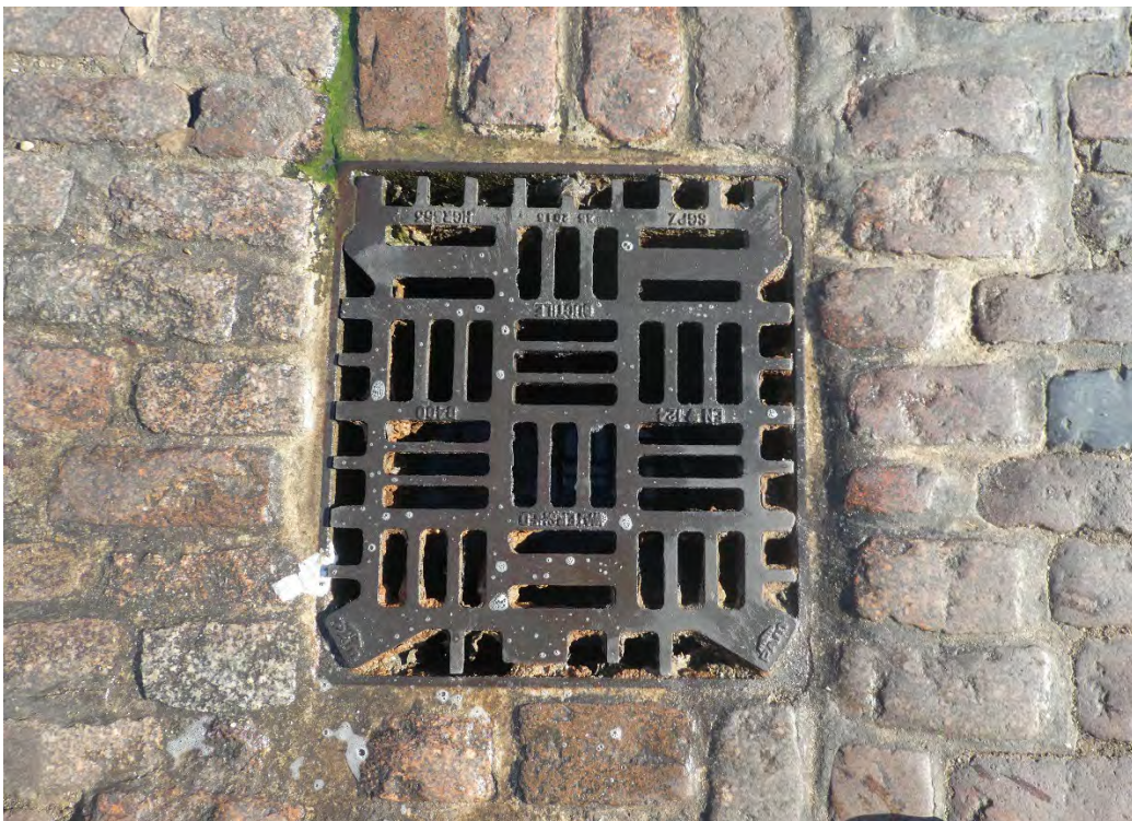
Photo 15: A drainage grating in zone 11 with 20mm wide slots.
