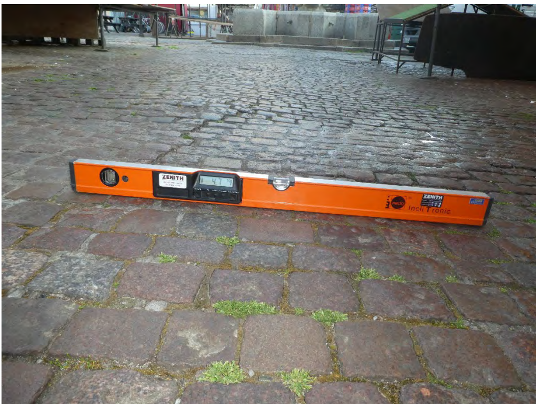
Photo 7: Walkway in zone 3 showing cross falls of 1 in 21.
