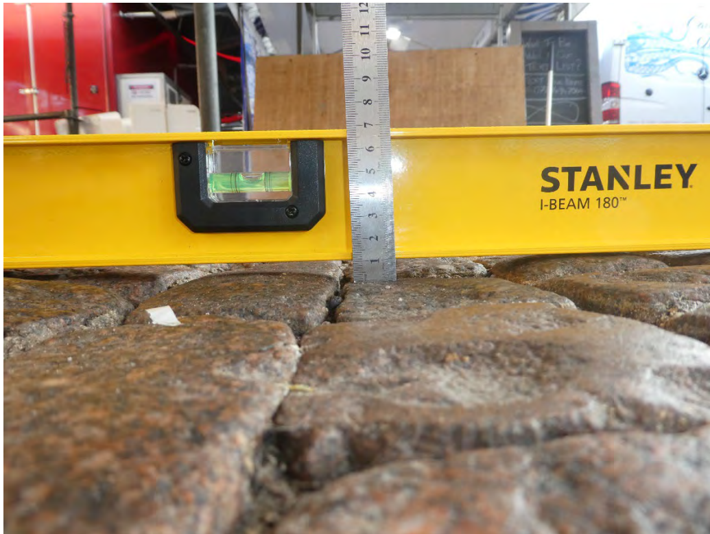
Photo 28: Example of how rounding of setts creates undulations, zone 2.
