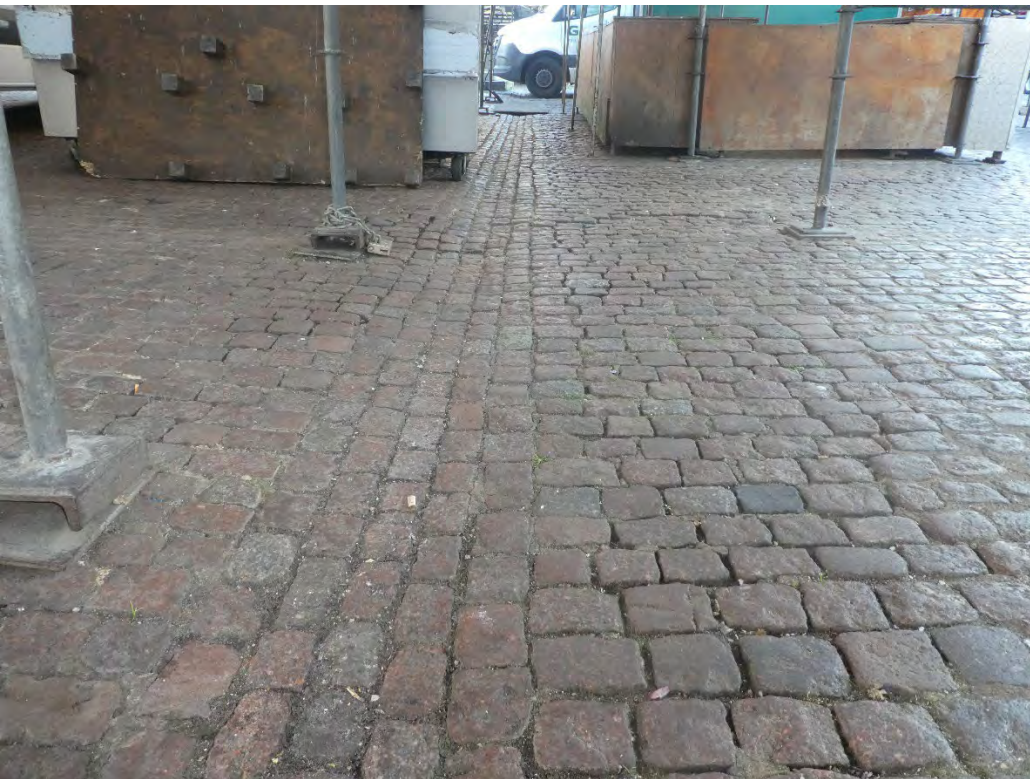
Photo 11: A 5 sett wide open channel running between rows of stalls.
