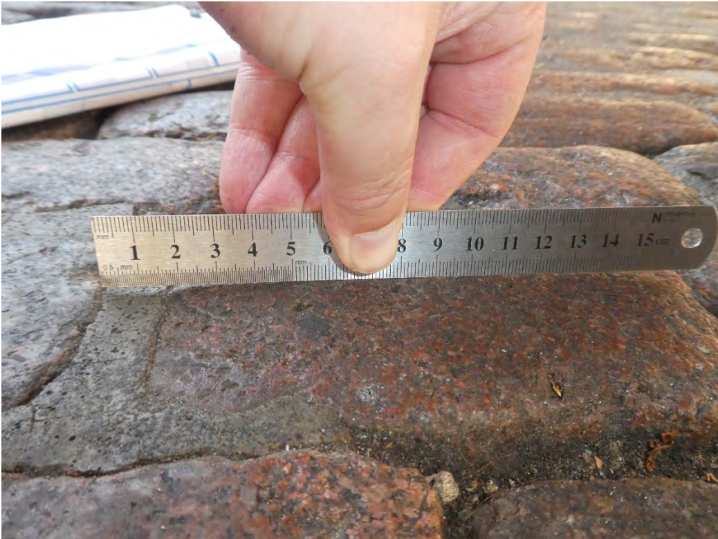
Photo 22: Example of one of the flatter setts with rounding to the edges.
