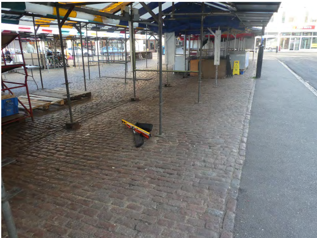
Photo 9: Zone 10 example showing falls to open channel between stalls.
