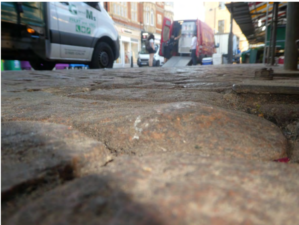
Photo 23: Example of one of the more rounded setts in zone 10.
