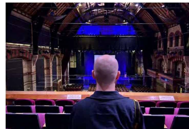
Balcony level sightlines are very poor as the rake is not steep enough and the seats are not staggered.
