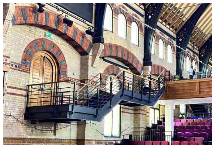
Escape stair is visually obtrusive within the space.
