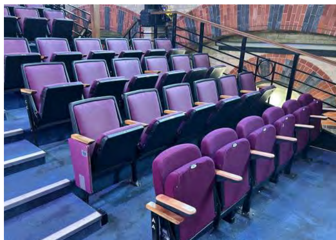
The balcony has not been sensitively inserted in relation to the period windows. The photo above also shows the mismatched seats.
