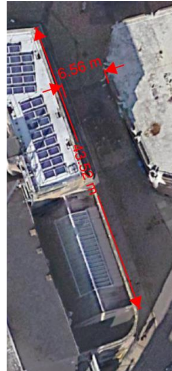
External fire spread measurements (representative of the closest boundary) © Google Maps
