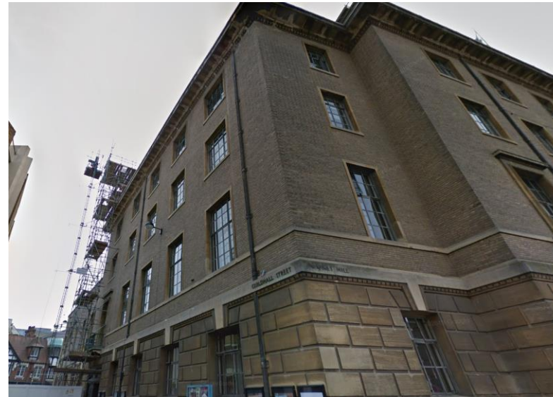
Guildhall external wall © Google Maps
