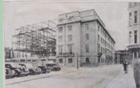
The second phase during construction in 1938
