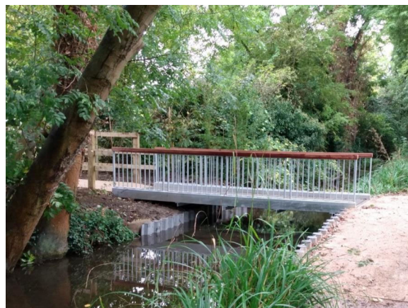
Footbridge over Hobson's Brook at Accordia development (2019/20)
