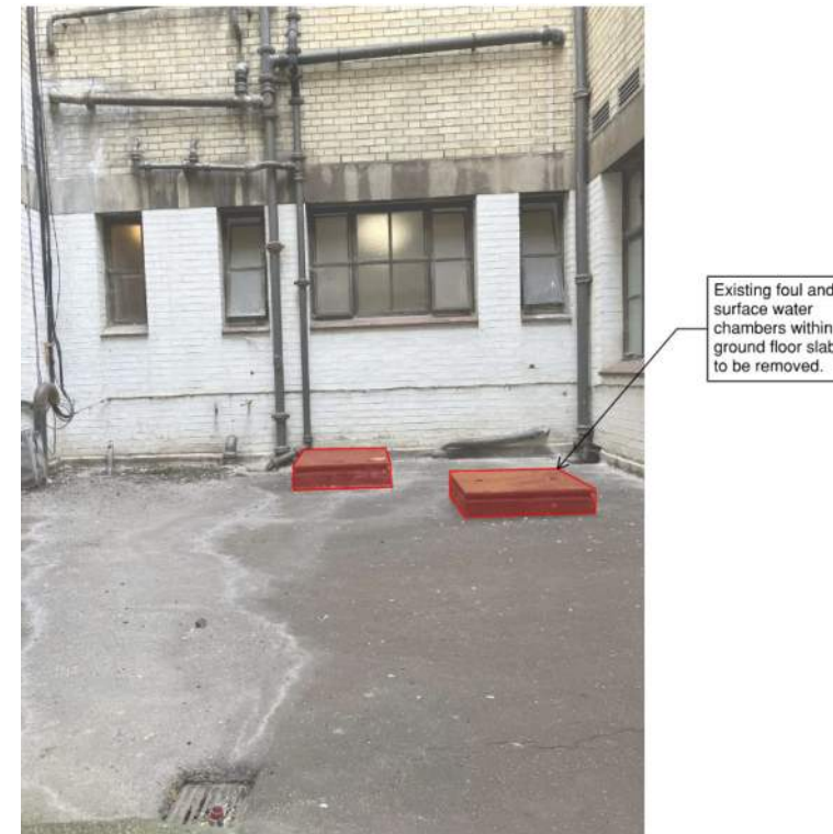
Existing chambers within ground floor slab to be removed
