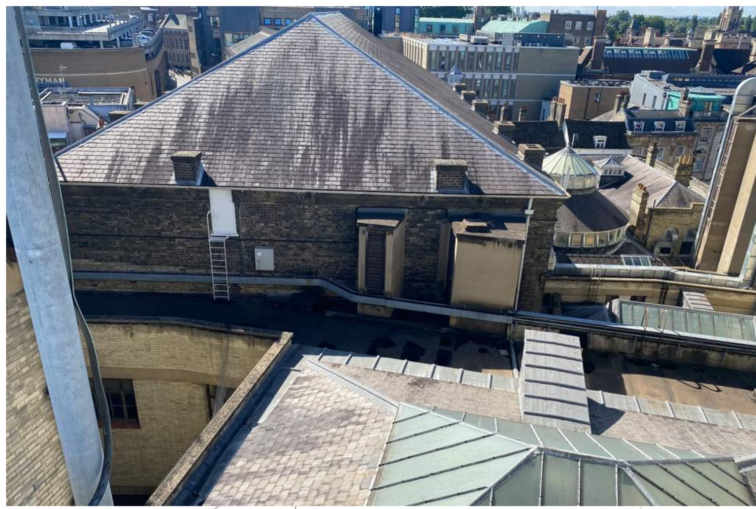
PHOTOGRAPH OF CHAMBER ROOF AND REAR OF LARGE ROOM
