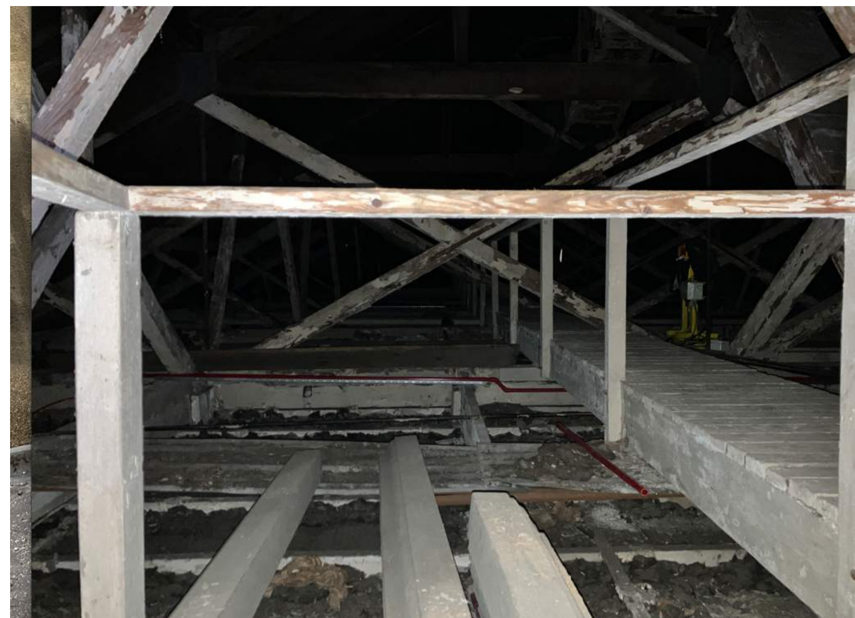
PHOTOGRAPH OF ROOF VOID ABOVE LARGE ROOM
