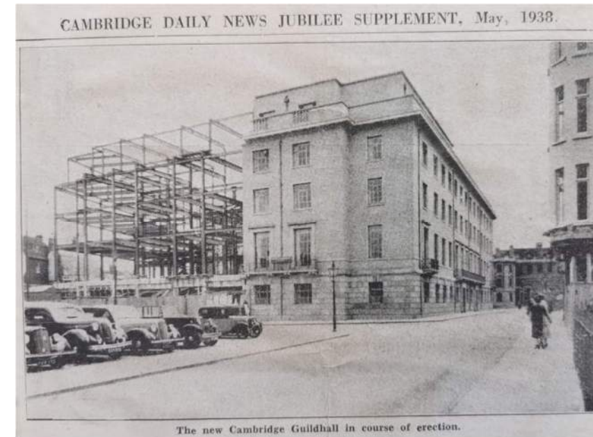
Central and eastern sections of Guildhall under construction 1930s
