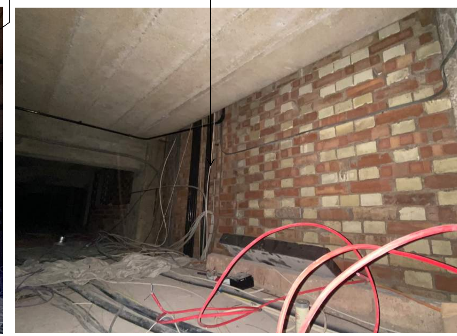
PHOTOGRAPHS SHOWING THE VOID ABOVE INSITU CEILING & EXISTING PRECAST FLOOR BEAMS AND ENCASED STEELWORK ABOVE
