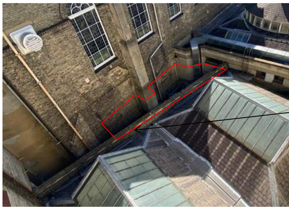
PHOTOGRAPH LOOKING DOWN FROM WESTERN ROOF
