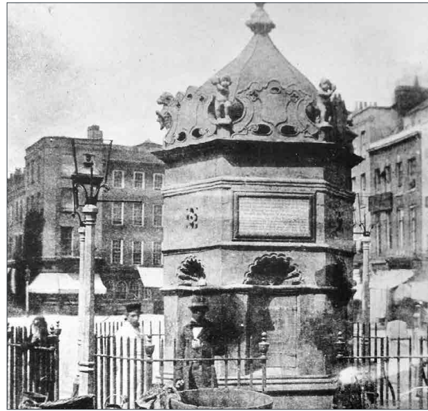
From 1614 - 1856 The Market Place branch of Hobson's Conduit was completed in 1614. This branch brought fresh water to the market fountain in the centre of the previous Market Place.
