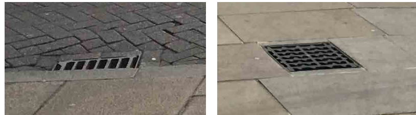
Bottom of kerb gully and gully on pedestrian area
