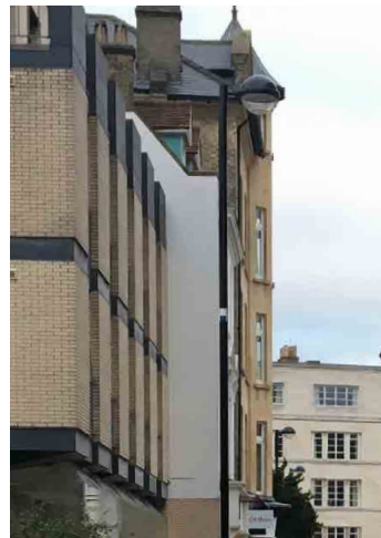
Single lighting posts DW Polar 500 Lantern 140W CPO-TW Lamp 8m high- RAL 9005 (Jet Black)
