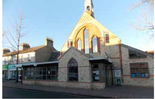
Figure 25: Photo ③ St Philip's Church and Community Centre, Mill Road
