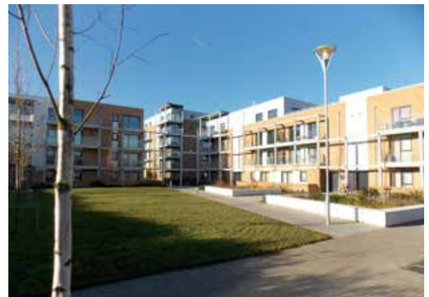
Figure 34: Photo ⑫ Pym Court on Cromwell Road
