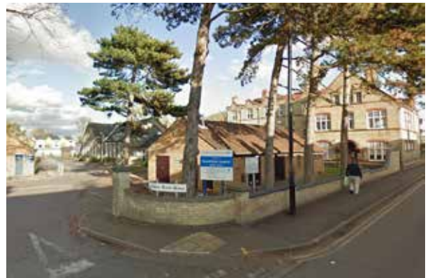
Figure 26: Photo ④ Brookfields Hospital, Mill Road
