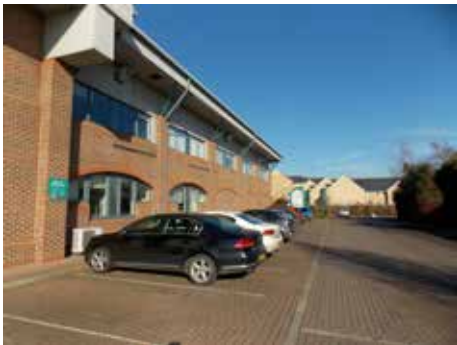
Figure 6: Photo ② Looking north on east side of showroom
