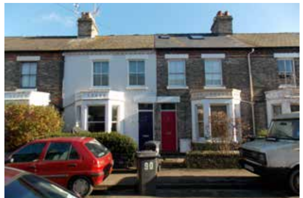
Figure 30: Photo ⑧ Terrace house on Cavendish Road, front garden and bay window
