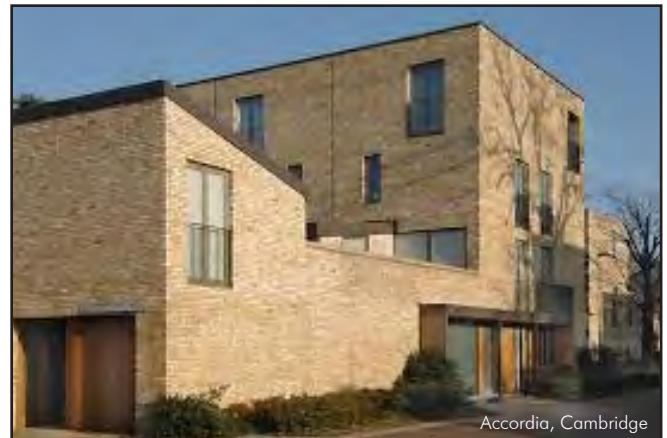
Figure 46: Well proportioned volumes and gaps creates a harmonious relationship between 4 storeys and 2 storey forms.
