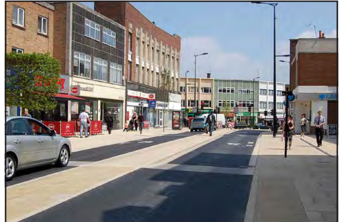
Figure 28: A reduced carriageway width, a central median strip and visual narrowing of the carriageway promotes lower speeds. (Hornchurch, London Borough of Havering).
