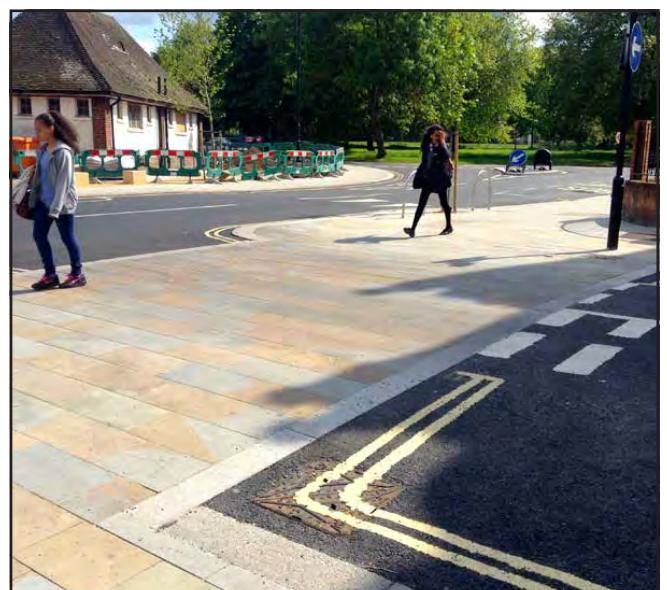
Figure 30: Extending footway treatment across side streets can help wheelchair users and people with prams move more freely and highlight pedestrian priority (London Borough of Lambeth)
