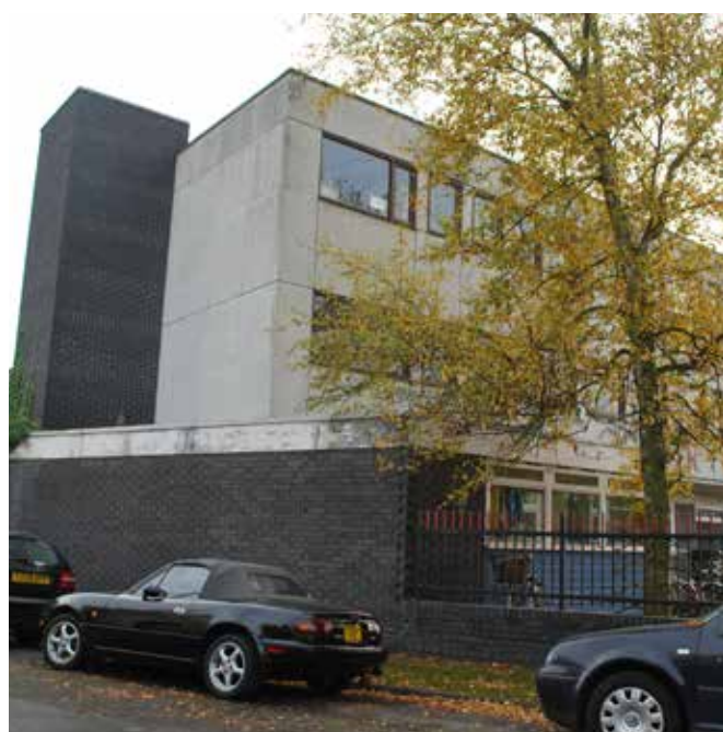
Fig 10 Existing site photographs. Above: The garages are situated at the northern end of the site adjacent to Hooper Street. Below: Women's Resource Centre
