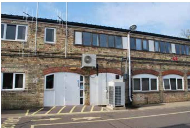
Fig 41 Above - adjacent to the Magna development, the old Rattee & Kett building has been converted to café/cookery school. This could be a relevant precedent for the coach houses on Mill Road (below)
