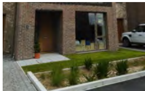
Bio-retention planter, Bell School Cambridge
