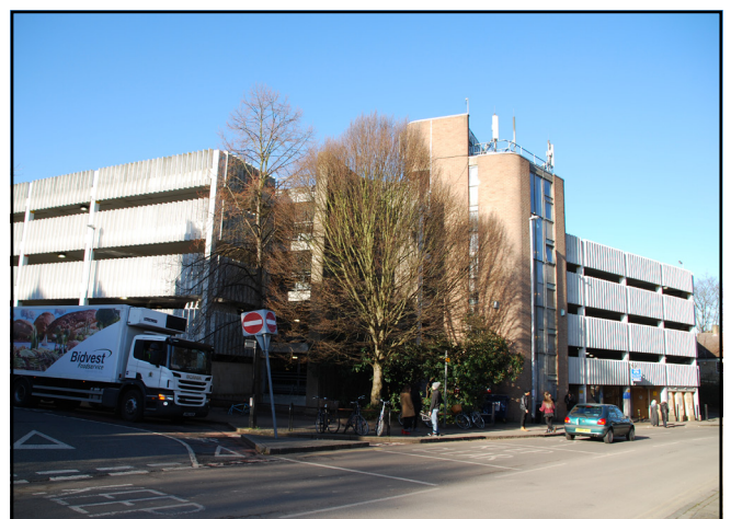
Figure 1: View of Park Street Car Park looking north-west
