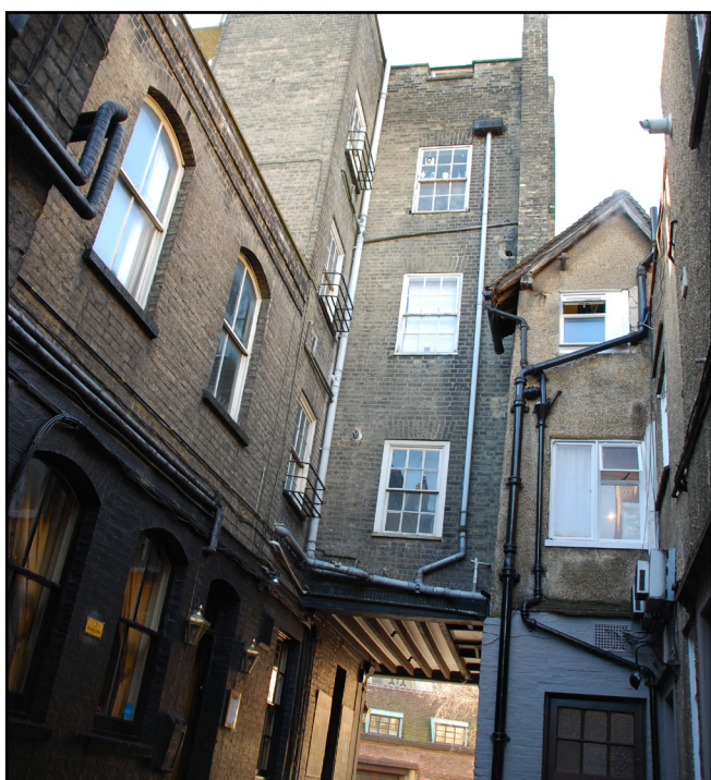
Figure 17: View from Blackmoor Head Yard looking towards Bridge Street
