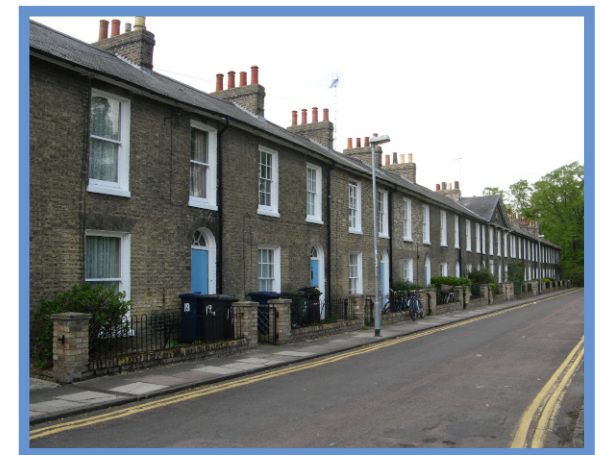
Terraced houses in New Square, South side
