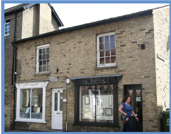
Shopfronts to Nos. 13 and 14 Fair Street
