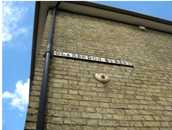
Cast iron nameplate on No. 40 Clarendon Street
