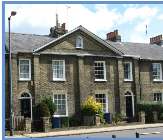
Houses in New Square
