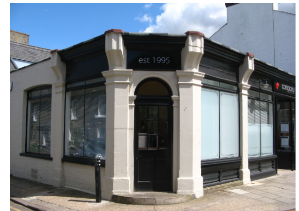
Single storey commercial building dating to c. 1925 in the Art Deco style which has been occupied by The Company Hairdressers since 1995. Flat roof with lead sheet dressings at the perimeter. Ogee section timber cornice above painted timber entablature. Projecting rendered pilasters with capitals and
