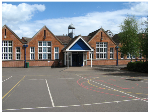
Very large, symmetrical single storey purpose-built school dating to the early 20th century – the former Boys Section facing Melbourne Place is dated 1912. The building sits back from Parkside on a rectangular backlands plot and is built in the Arts and Crafts style with red brick facings, gables, timber windows and hipped tiled roofs. The plan form appears to be virtually unaltered with a courtyard
