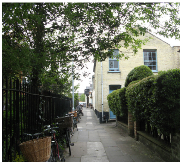
Melbourne Place poor paving
