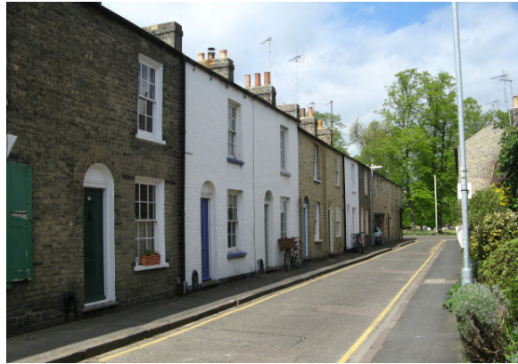
Circa 1841. Grey Gault brick. Two storeys, one window, sashes with glazing bars. Panelled doors with arched heads.
