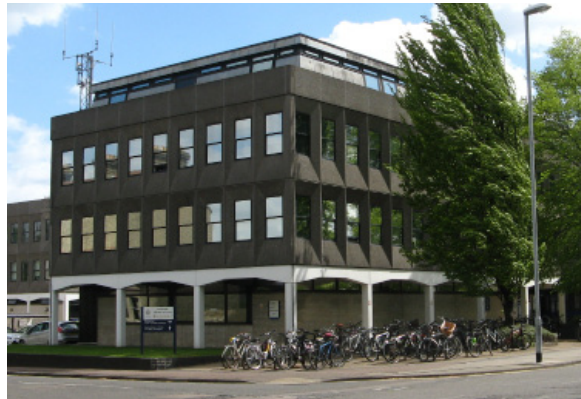
This substantial L-shaped four storey building is nine bays long and three bays deep, with a back extension of a similar size and details, set well back from Warkworth Terrace. It is built from dark brown brick with a colonnade to the ground floor supported on contrasting
