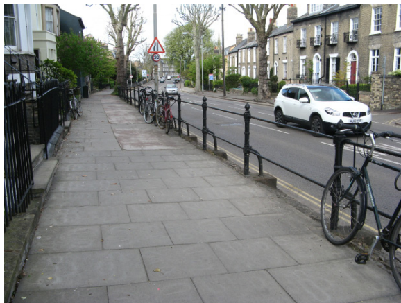
Raised pavement in Maids Causeway
