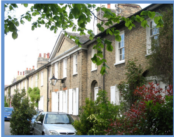
Raised pediment over Nos. 9 and 10
