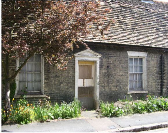
No. 7 Orchard Street is a Building at Risk
