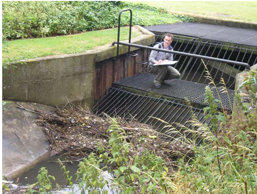
Figure B5.2: Milton Road Siphon
