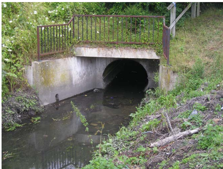
Figure B2.2: East Cambridge Main Drain passing under Newmarket Road
