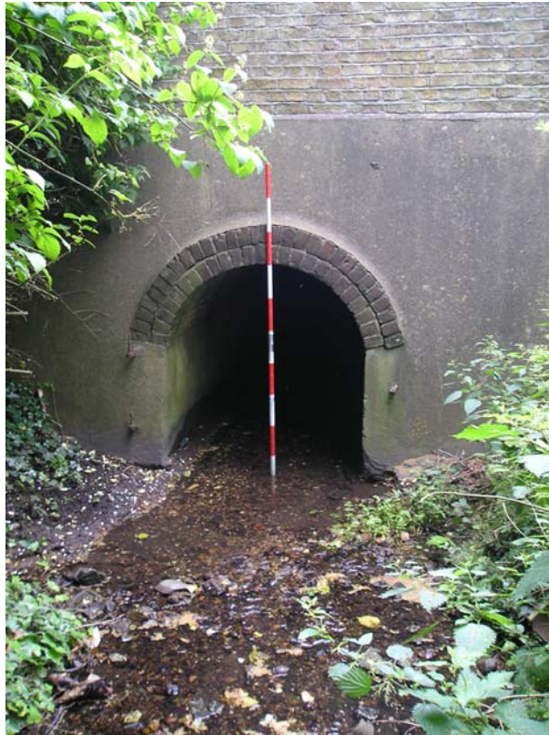
Figure B4.3: Vicar's Brook Culvert under Trumpington Road
