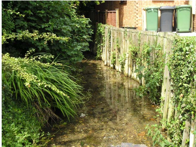
Figure B1.2: Property on Right Bank Downstream of Forest Road Culvert
