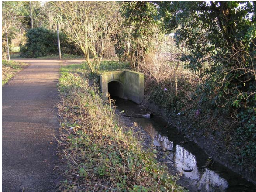
Figure B7.2: Daws Lane Ditch, Upstream Extent
