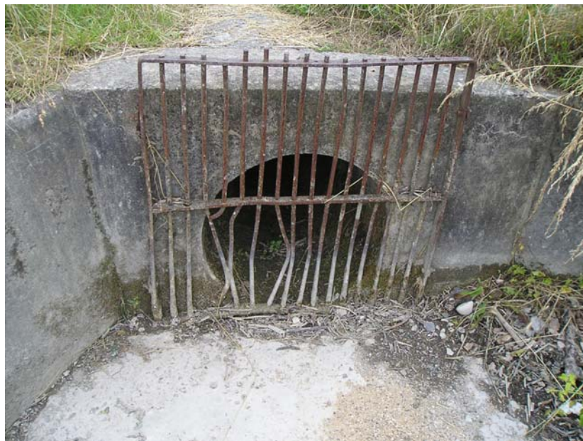
Figure B1.4: Dry Culvert on Coldham's Common
