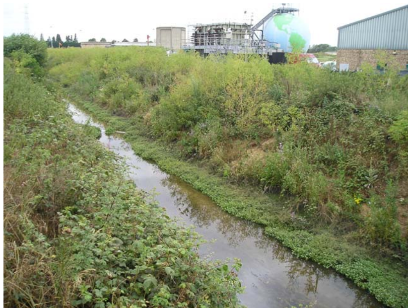
Figure B5.4: First Public Drain alongside Cambridge Wastewater Treatment Works
