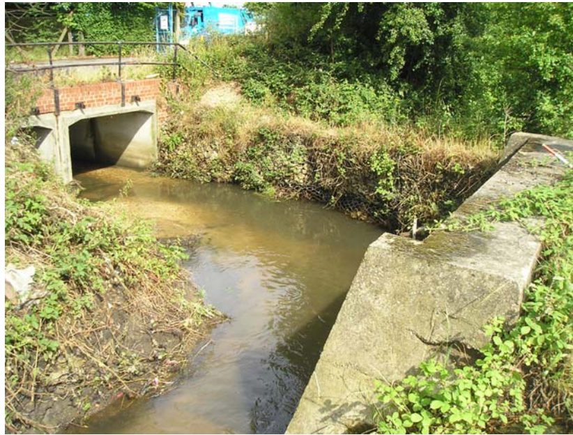
Figure B5.3: Cowley Road Bend and Culverts
