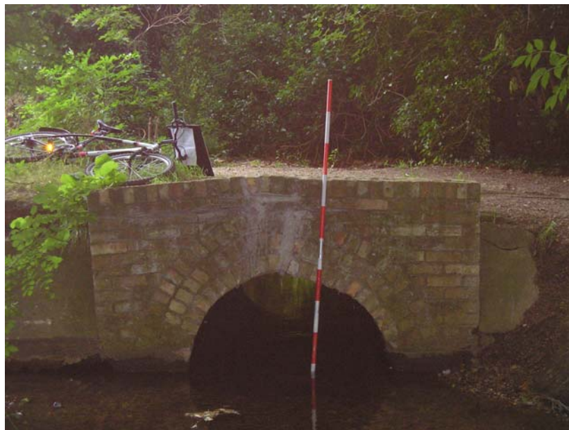
Figure B4.4: Bridge at End of Porson's Road
