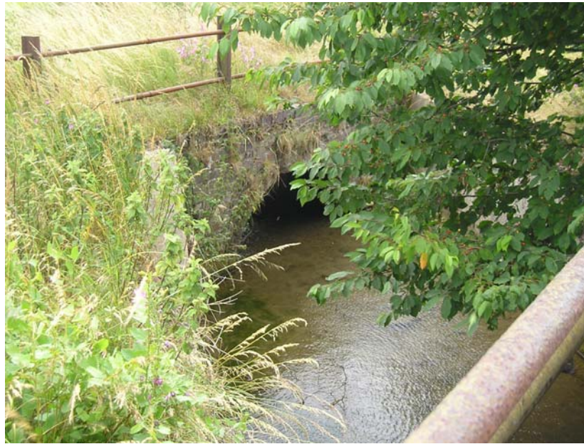
Figure B4.2: Disused Railway Bridge
