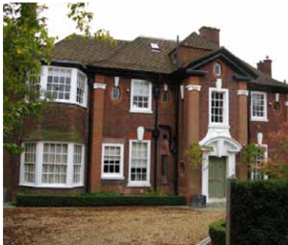
No. 1 Latham Road
