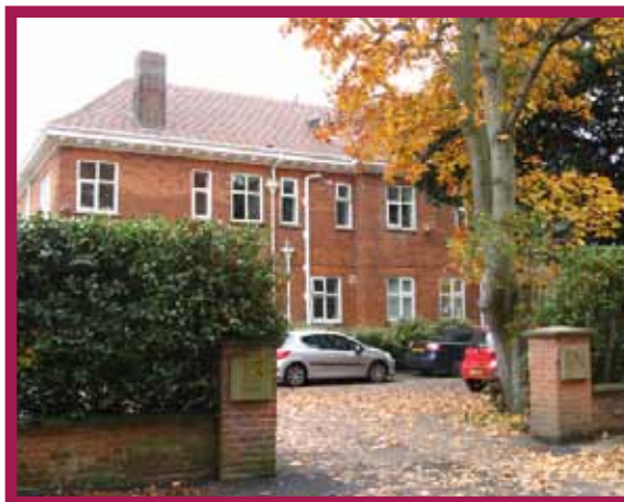
MRC Unit at No. 15 Latham Road
