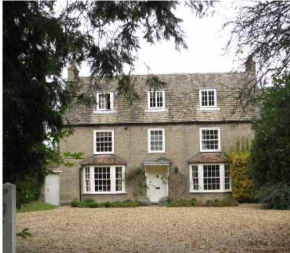
No. 10 Latham Road and attached garage/studio, Grade II (spot listed in 1999)
