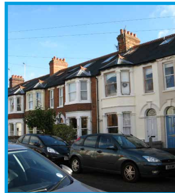
Nos. 1-32 (conseq.) on the south-east side of Eltisley Avenue
