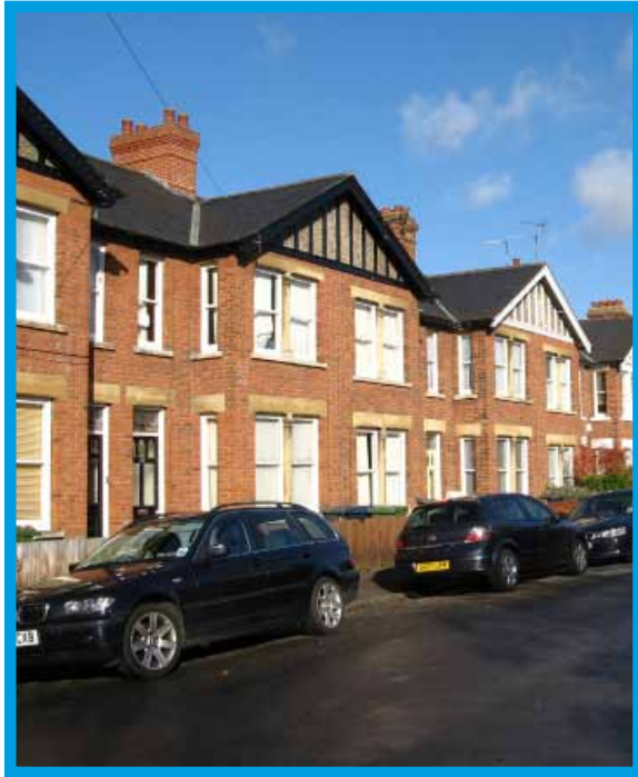
North west side of Eltisley Avenue
