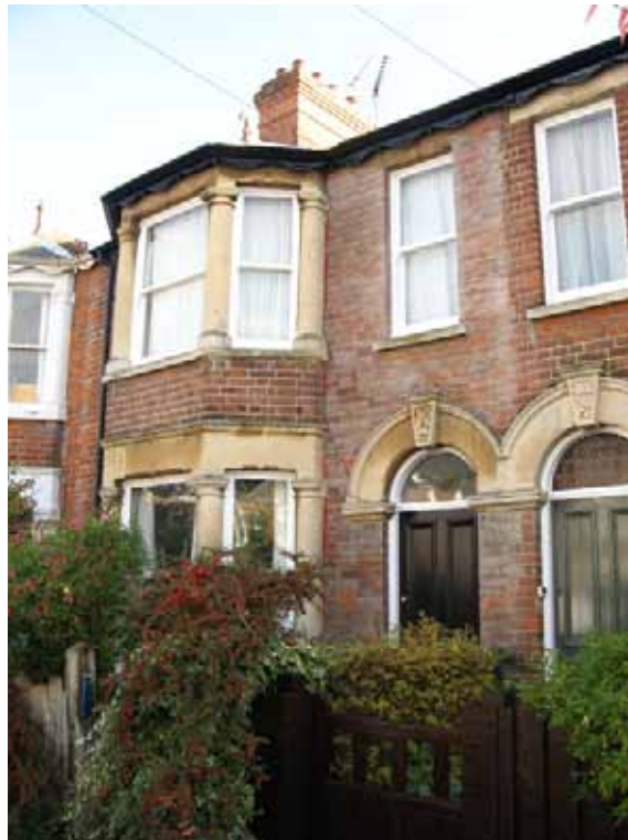
Detail of house to south east side of Eltisley Avenue
