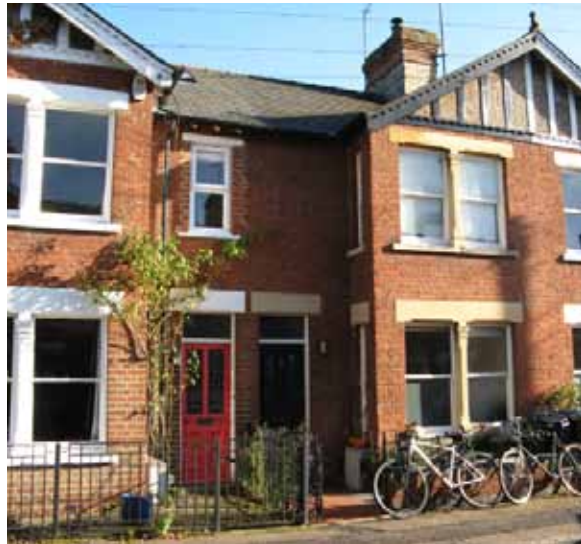
Detail of a Marlowe Road house
