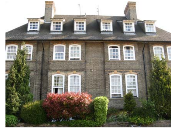
Nos. 1 and 2 Wollaston Road
