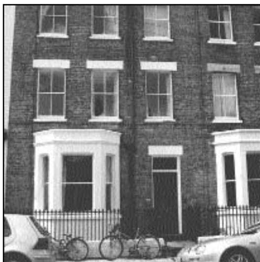
Basements provide extra accommodation without using more land.
