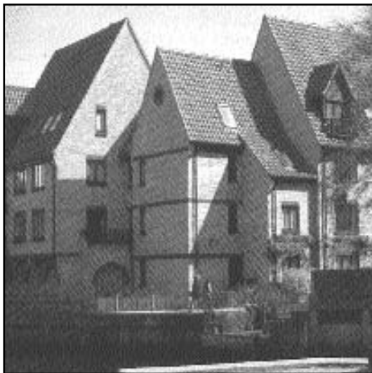
Well designed corner buildings such as these in Norwich add visual interest, avoid wasted space and can help integrate new development into the surrounding area.
