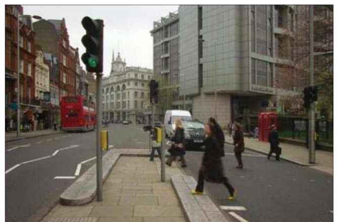
Figure 52: Crossings have been redesigned with the removal of guardrails (Kensington High Street, London)
