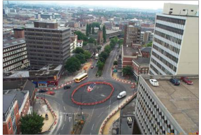
Figure 45: Filling in the subways with concrete
