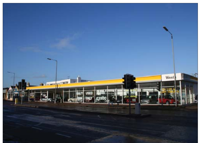
Figure 23: Poor quality warehouse and car showroom buildings create barriers to movement between residential areas north and south of Newmarket Road
