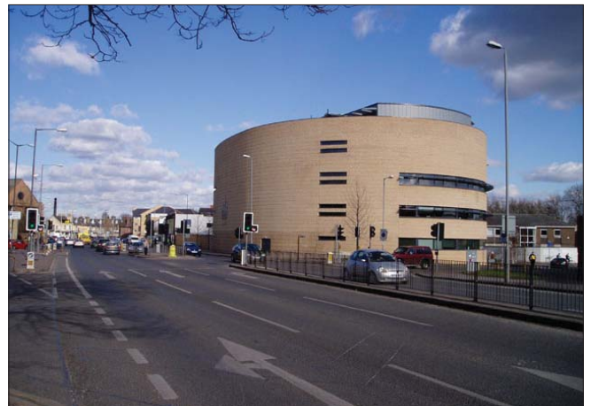
Figure 26: View of Cambridge Crown Court, looking north-east along East Road
