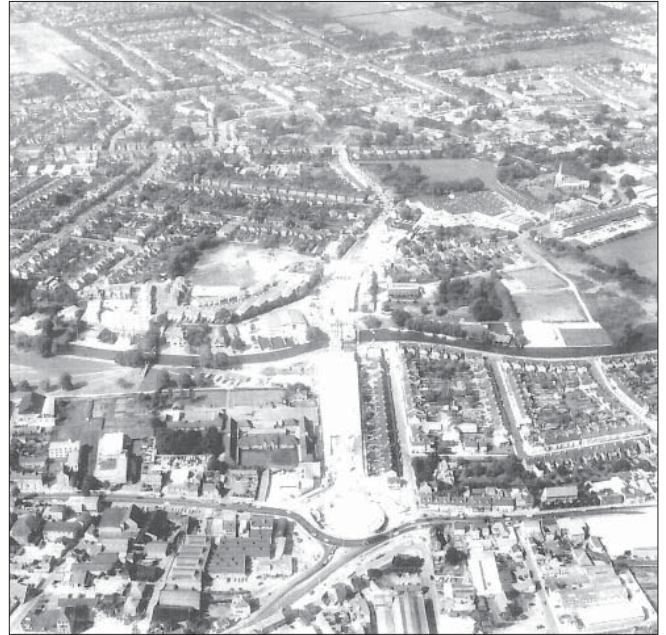
Figure 7 (above) and Figure 8 (right): Photographs showing the construction of Elizabeth Way Bridge in 1971
