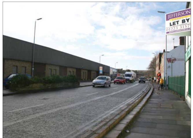
Figure 22: poor quality and passive frontages create hostile and uncomfortable edges
