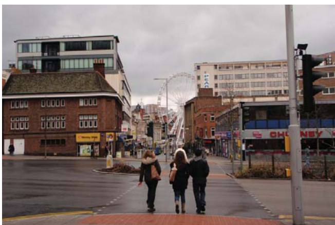
Figure 51: Wide, direct, pedestrian crossings redesigned to respond to key desire lines and located close to the junction - note the absence of pedestrian guardrails (Maid Marion Way, Nottingham)
