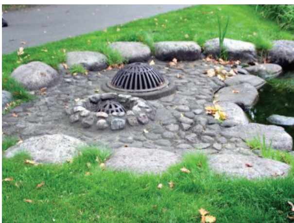
Overflow outlet from a pond
