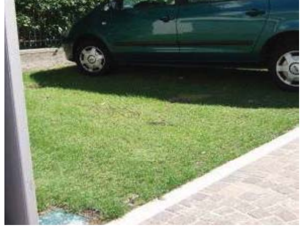
Reinforced grass car park surface, Lake Garda, Italy
