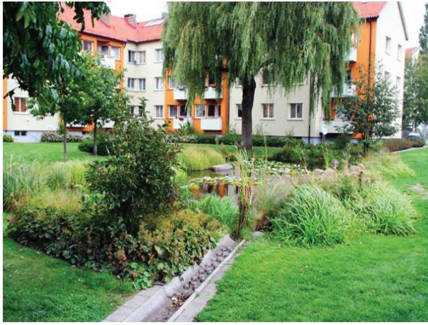
SUDS integrated into urban design provide a high quality urban environment, Malmö, Sweden
