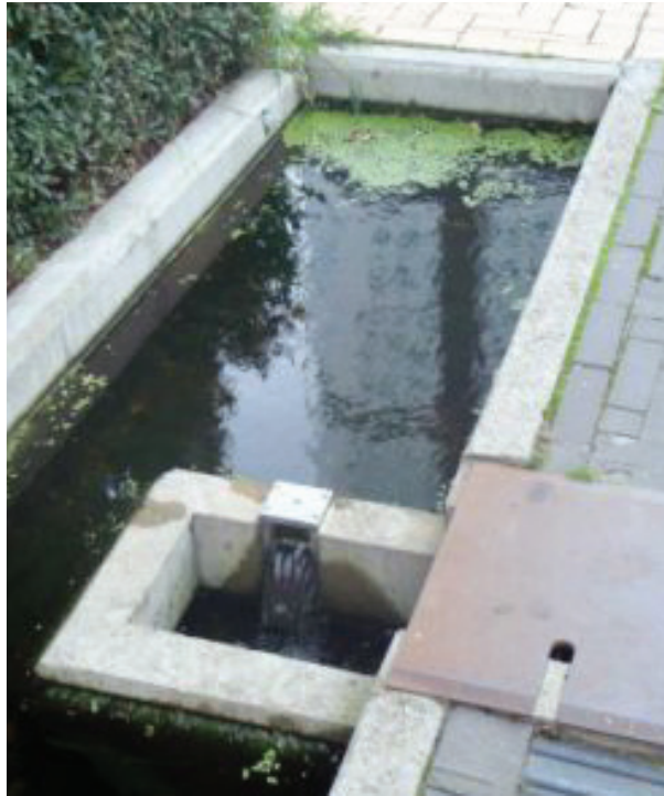
Outlet from a small urban SUDS water feature
