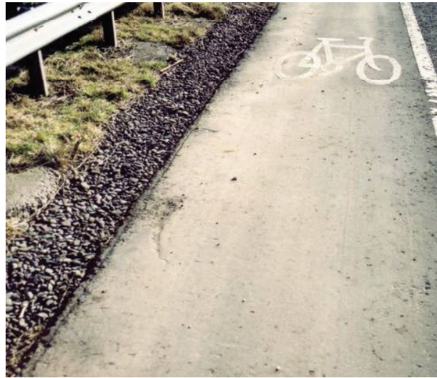
Road side filter drain, A74, Scotland
