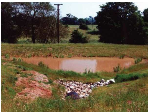
Silt in a pond during construction caused by erosion due to lack of topsoil and vegetation, motorway service area, M42
