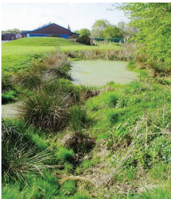
Algae in a SUDS pond is common in the first year or two after construction, Worcestershire
