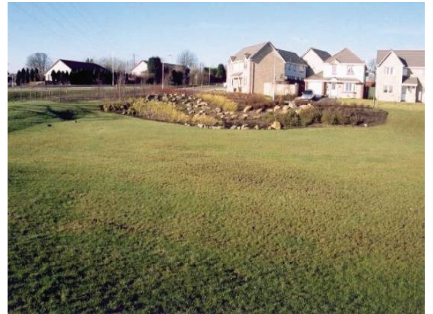
Shallow retention basin with easy access for maintenance, forming part of the public open space for the development
