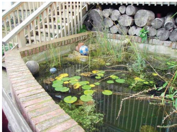
Small SUDS pool in high density housing – due to the close proximity to buildings hard edges are appropriate in this development, Stroud, Gloucestershire
