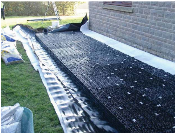
Rainwater harvesting tank being constructed below a patio, Derbyshire
