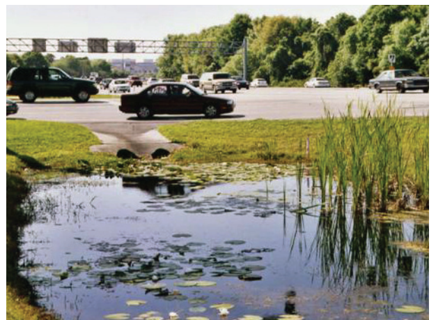
Shallow pond with gentle side slopes provides a safe feature with easy access for maintenance, Florida, USA
