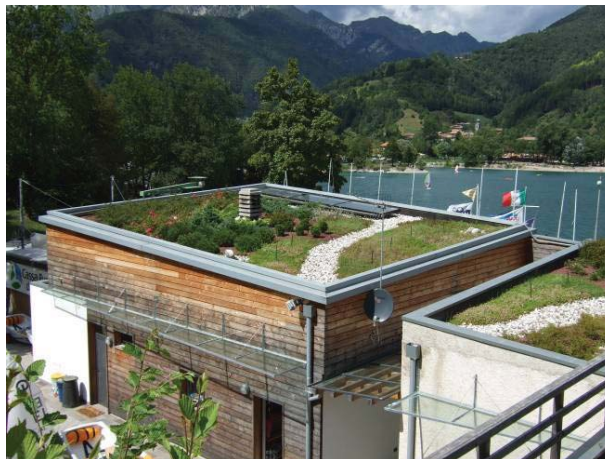
Green roof on a community building, Lake Ledro, Italy
