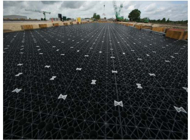
Shallow geocellular storage used below permeable paving as a subbase replacement at a Park and Ride site in Cambridgeshire
