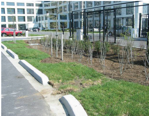
Recently constructed rain garden (bio retention) in a car park, Maryland, USA
