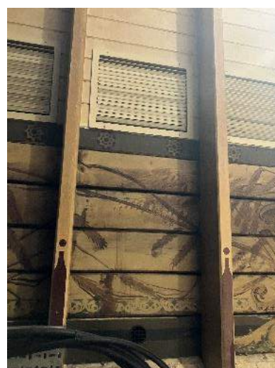
Auditorium high level supply grilles. Linear above timber slats, circular in metal panel under.
