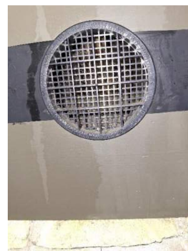
Auditorium high level supply grilles. Linear above timber slats, circular in metal panel under.
