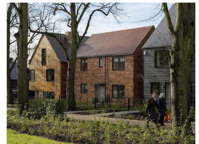
Entrances visible from public spaces, The Avenue, Pollard Thomas Edwards
