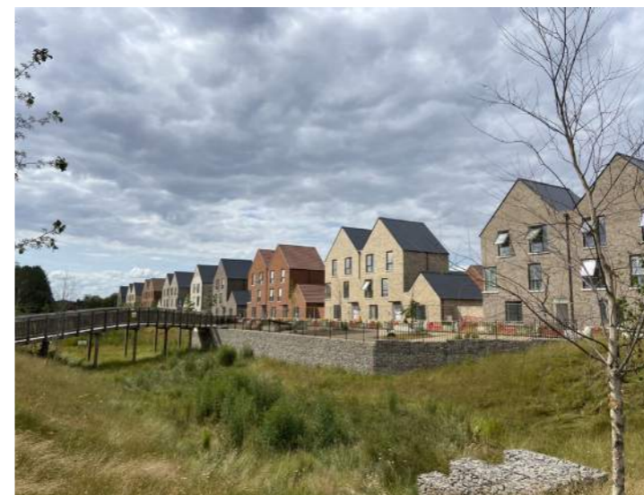
Houses looking over landscape with SUDs. Services hidden away at the rear. Marleigh, Pollard Thomas Edwards
