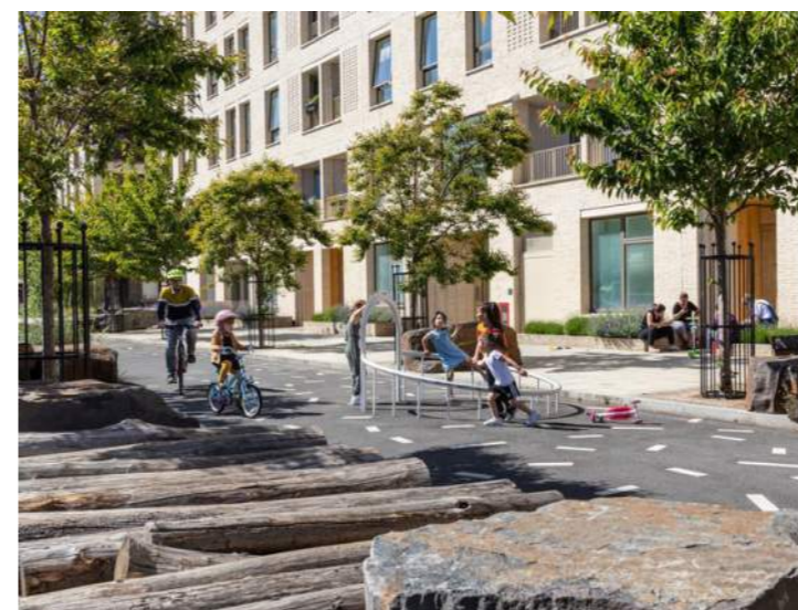
Improving key active travel routes, Kings Crescent Estate, Hackney Council, Henley Hale Brown
