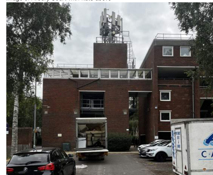
Photograph of a flat block in Arbury, with a service bay being the predominate vista
