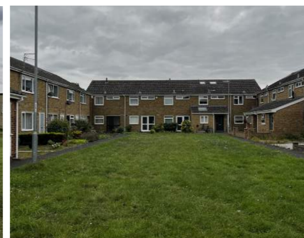
Image of a green courtyard
