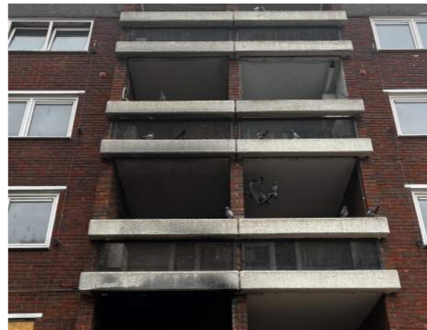
Image of a flat block deck access
