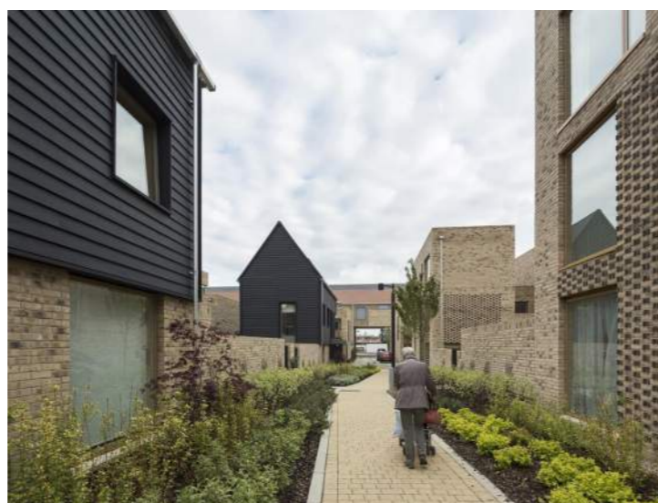
Making routes attractive through planting and lighting, Abode, Cambridge, Proctor Mathews
