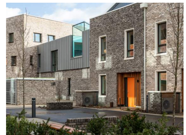
Screened ASHP integrated into Public-Realm, Marmalade Lane , William Green Architects
