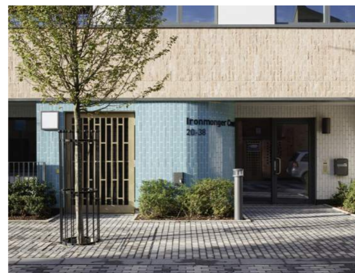
Thoughtful integrated cycle stores that are secure and found close to entrances, Charter Place, Hounslow Council, Pollard Thomas Edwards
