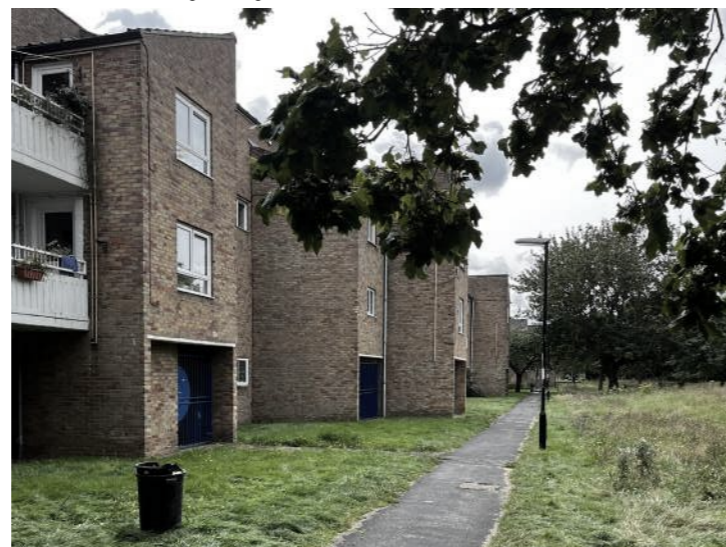
4. Front elevation facing onto a green open space
