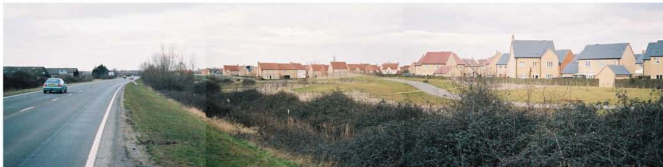
A10 by-pass around Ely, with recent residential development. A linear public space has been created between the busy road and new housing. The distance from the road boundary to the closest houses varies between 50 - 75 metres. Extensive tree planting will hopefully mature into a screen between the road and estate and the space will become a 'woodland walk'. However it is expected that this scale of landscape space will be perceived as having an 'urban' character. 'Ely' will extend to the road edge.
