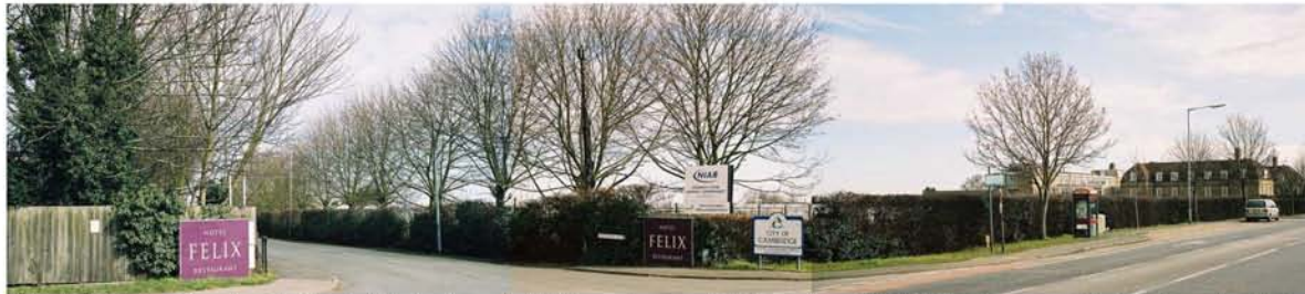
View 14 looking south-east on Huntingdon Rd at entrance to Whitehouse Lane and NIAB premises. This NIAB land is proposed for development - although the main buildings beyond are proposed for retention.
