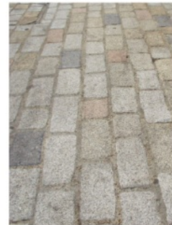
Sensitive paving, Somerset House
