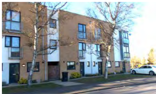
Figure 87: 3 storey houses in the Pym Court development on Cromwell Road
