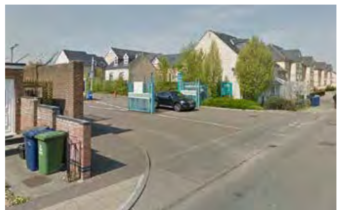
Figure 117: Retaining the existing vehicle route into the site as the only vehicle entry point into the new development. Entrance should be narrowed.
