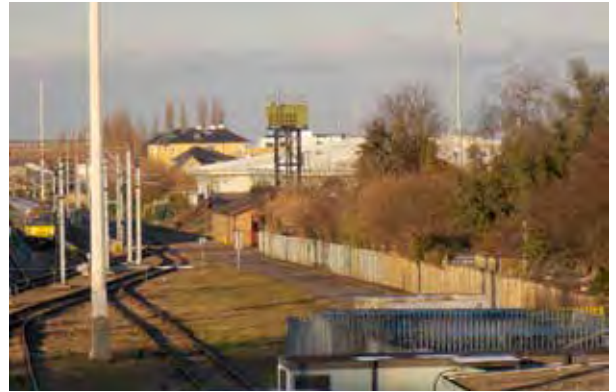
Figure 23: Photo ① View towards Ridgeons from Mill Road bridge
