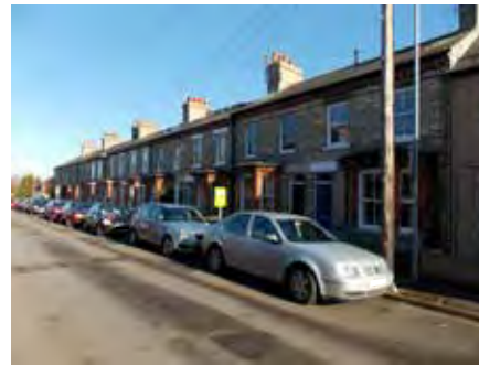
Figure 15: Photos ⑩ Houses on Sedgwick Street in Mill Road Conservation Area
