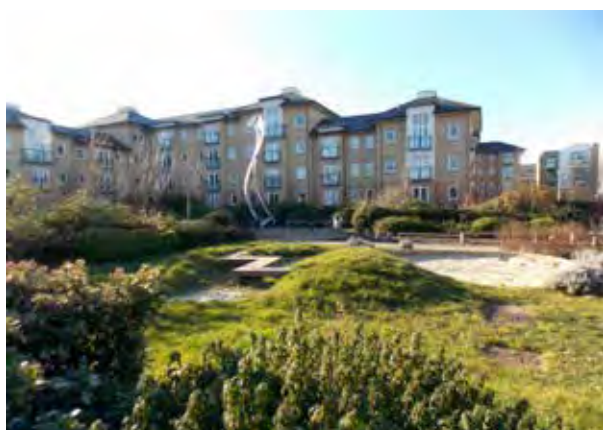
Figure 33: Photo ⑪ Park at Hampden Gardens on Cromwell Road
