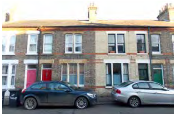
Figure 29: Photos ⑦ Terrace house on Catherine Street - no front boundary
