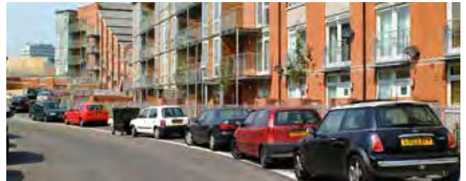
Figure 118: Parallel on-street bays
