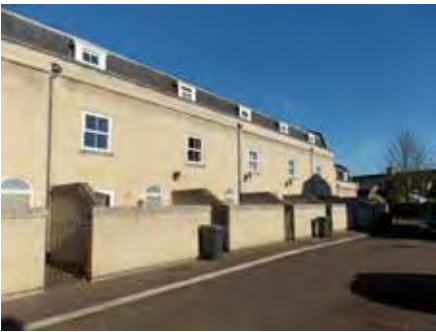
Figure 14: Photo ⑨ Terrace of houses to south of Ridgeons site
