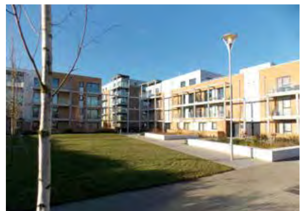
Figure 34: Photo ⑫ Pym Court on Cromwell Road
