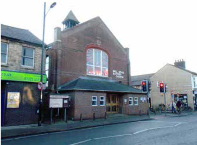
Figure 59: Mill Road Baptist Church
