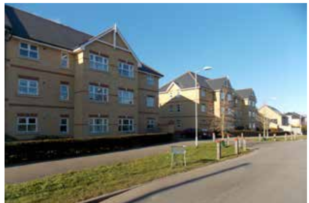
Figure 32: Photo ⑩ Winstanley Court on Cromwell Road
