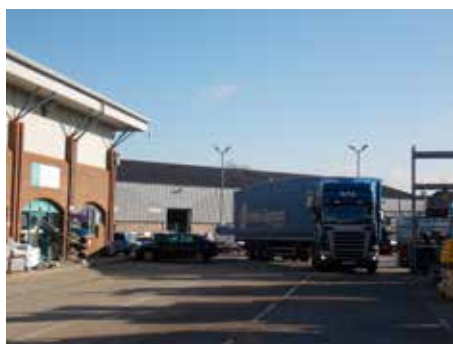
Figure 9: Photo ⑤ Looking east to south of timber and joinery warehouse
