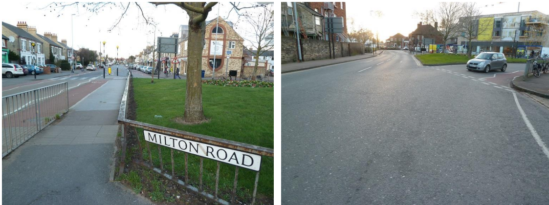
Significant areas of underused space and wide carriageway dimensions
