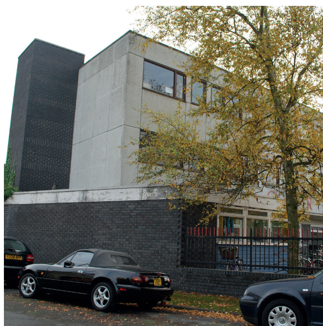
Fig 10 Existing site photographs. Above: The garages are situated at the northern end of the site adjacent to Hooper Street. Below: Women's Resource Centre
