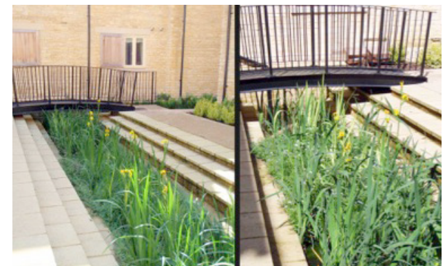
Planted urban conveyance rills (Robert Bray Assoc.)
