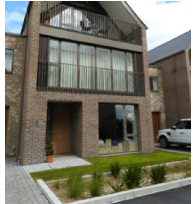
Bio-retention planter, Bell School Cambridge
