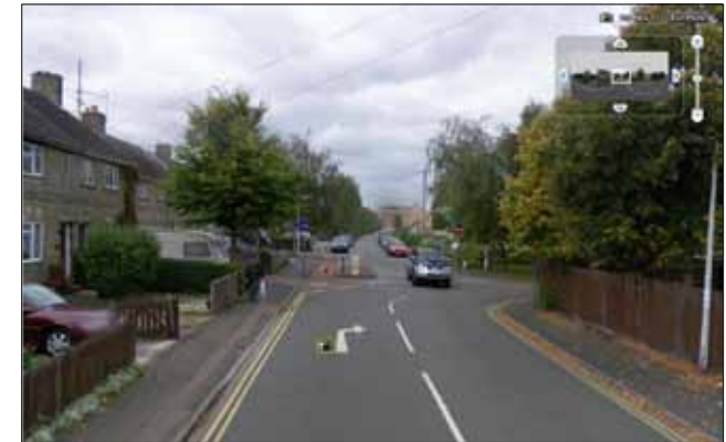
Figure 83: The existing situation... Uninterrupted views, wide carriageway widths and narrow footways, reinforce vehicle dominance. (View looking west along New Street towards Harvest Way junction)
