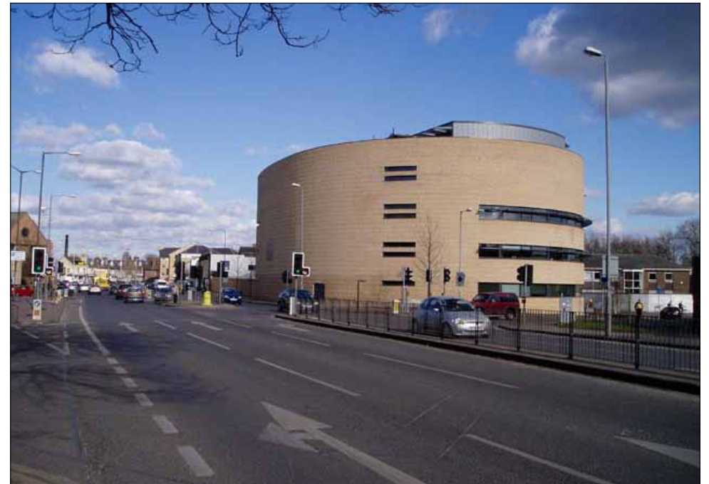
Figure 45: View of the Cambridge Crown Court, taken from East Road >
