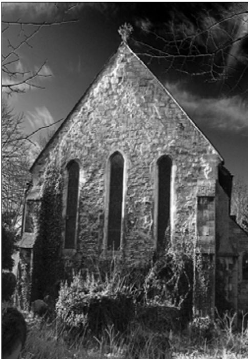
Figure 13: Photograph of St Andrew-the-Less (Abbey Church) showing the east gable (date unknown)
