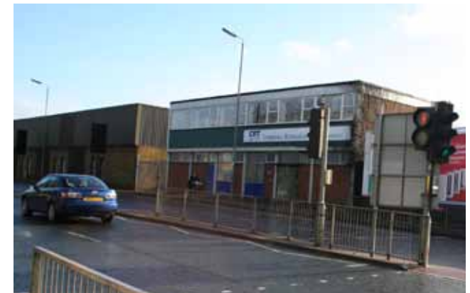
Figure 24: Pedestrian guardrails present barriers to movement.
