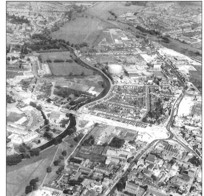
Figure 19 (above) and Figure 20 (right): Photographs showing the construction of Elizabeth Way Bridge in 1971
