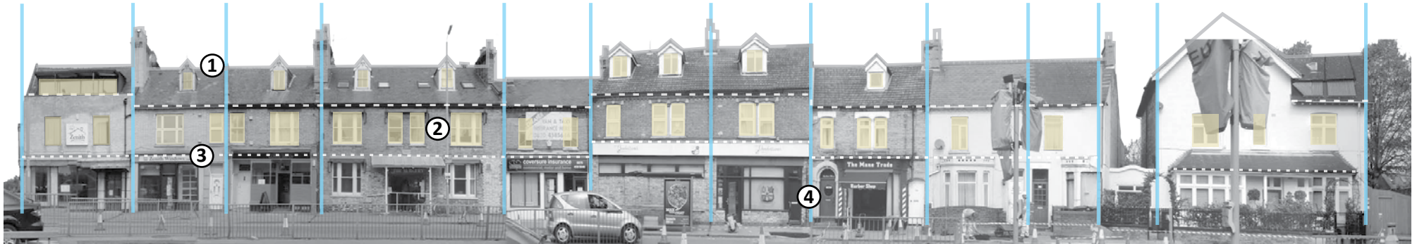
Figure 57: Key contextual elements - Newmarket Road frontage, east of Elizabeth Way roundabout (Top image: North side, middle Image: South side)
