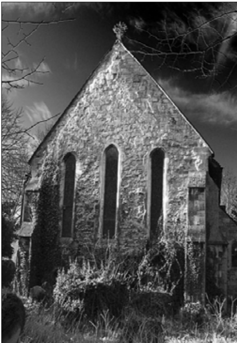
Figure 13: Photograph of St Andrew-the-Less (Abbey Church) showing the east gable (date unknown)
