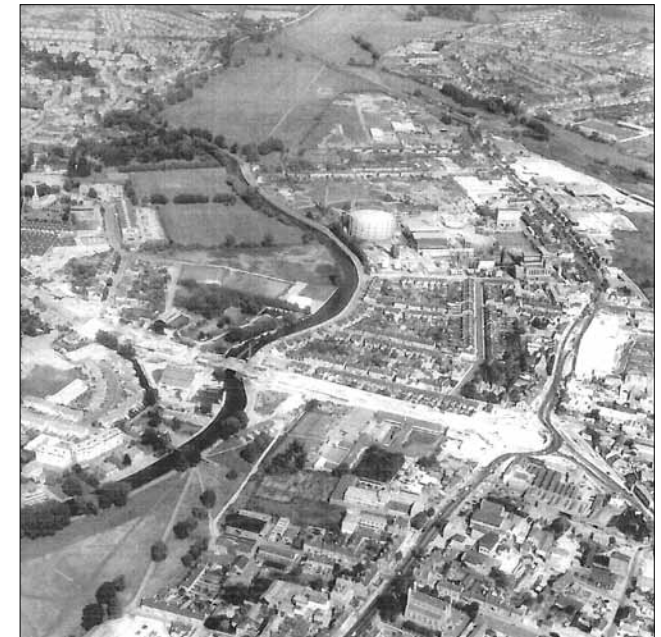
Figure 19 (above) and Figure 20 (right): Photographs showing the construction of Elizabeth Way Bridge in 1971
