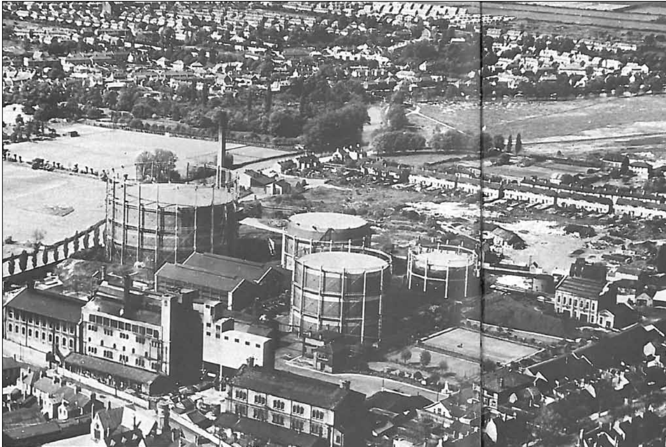
Figure 17: Photograph of the Newmarket Road Gas Works (Circa 1950)
