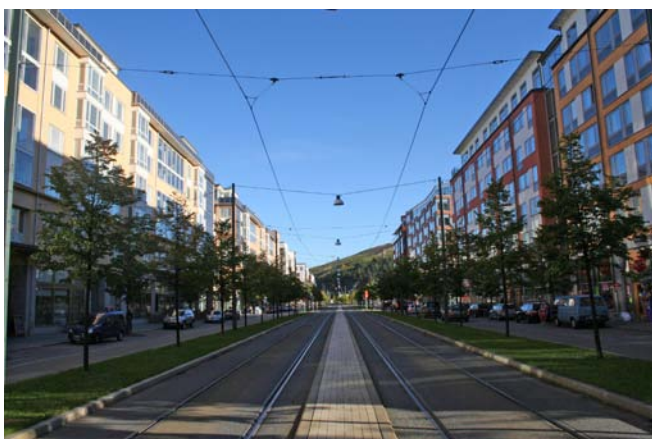
Figure 54: Central tramlines prioritise public transport movement. Median strips accommodate trees and allow for informal pedestrian crossings (Hammarby Sjöstad, Stockholm, Sweden)
