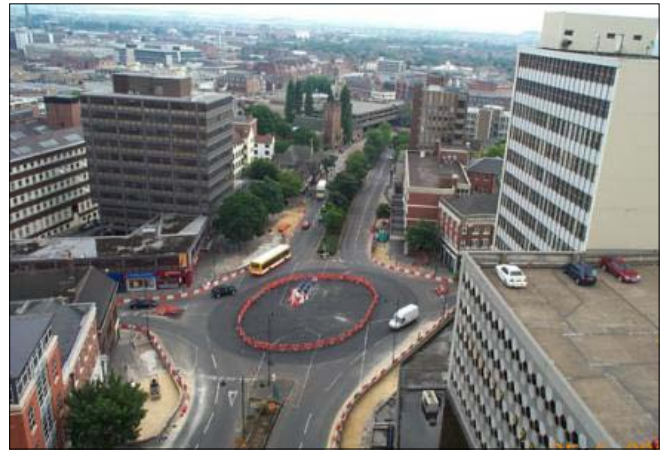
Figure 46: Filling in the subways with concrete
