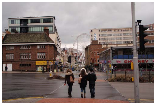
Figure 52: Wide, direct, pedestrian crossings redesigned to respond to key desire lines and located close to the junction - note the absence of pedestrian guardrails (Maid Marion Way, Nottingham)
