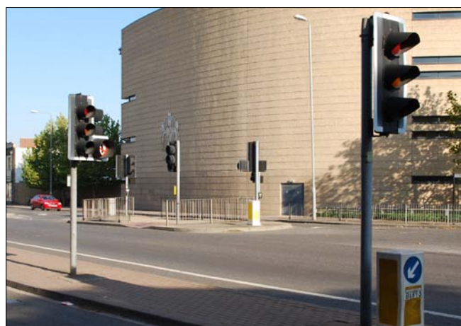
Figure 13: Pedestrian guardrails present barriers to movement
