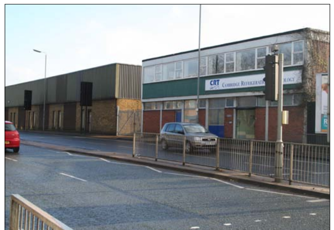
Figure 28: Large scale industrial buildings front Newmarket Road (view looking east along Newmarket Road).
