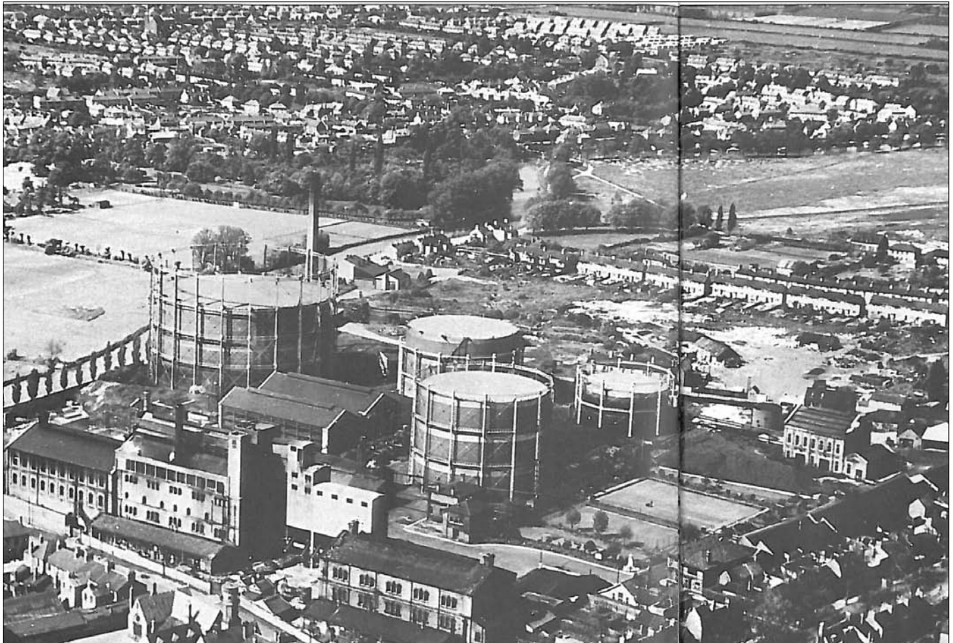
Figure 12: Photograph of the Newmarket Road Gas Works (Circa 1950)
