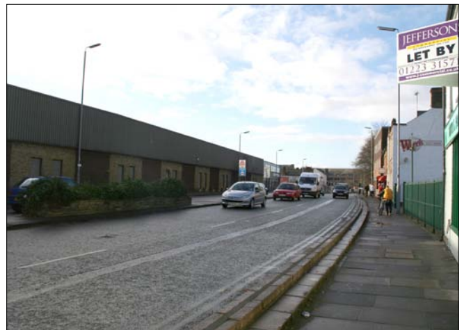
Figure 23: Poor quality and passive frontages create hostile and uncomfortable edges
