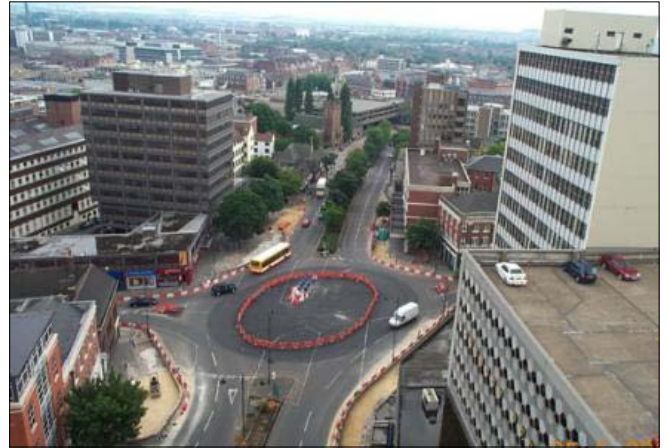
Figure 46: Filling in the subways with concrete
