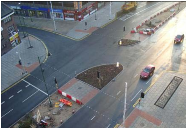
Figure 47: The roundabout after - signalised junctions
