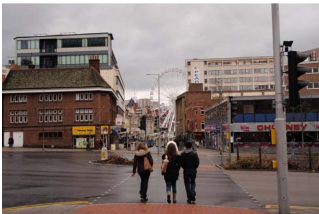
Figure 52: Wide, direct, pedestrian crossings redesigned to respond to key desire lines and located close to the junction - note the absence of pedestrian guardrails (Maid Marion Way, Nottingham)
