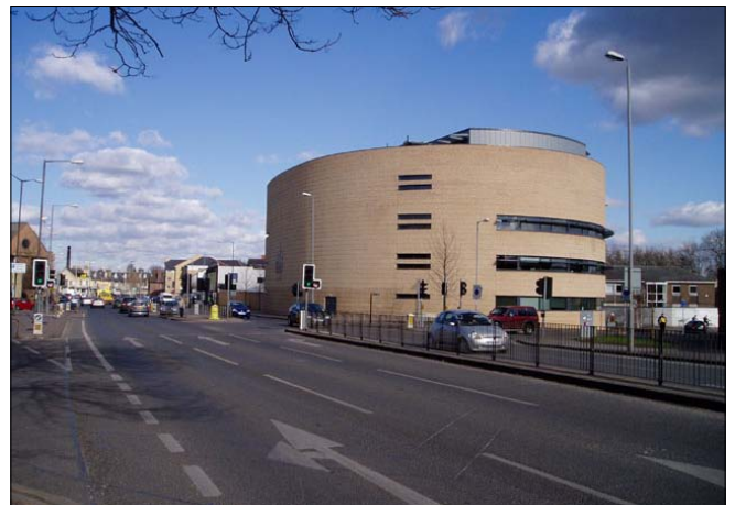
Figure 27: View of Cambridge Crown Court (looking north-east along East Road)
