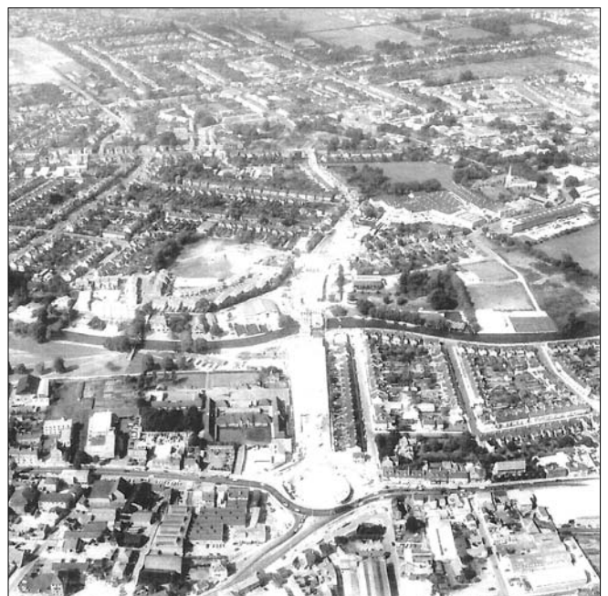
Figure 9 (top) and Figure 10 (above): Photographs showing the construction of Elizabeth Way Bridge in 1971
