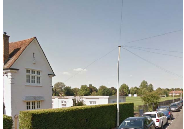
Figure 10 - View north from adjacent the Pavilion
