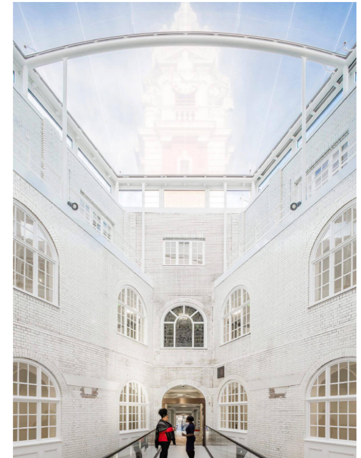
Lambeth Town Hall exemplar ETFE roof (Source: Cartwright Pickard)
