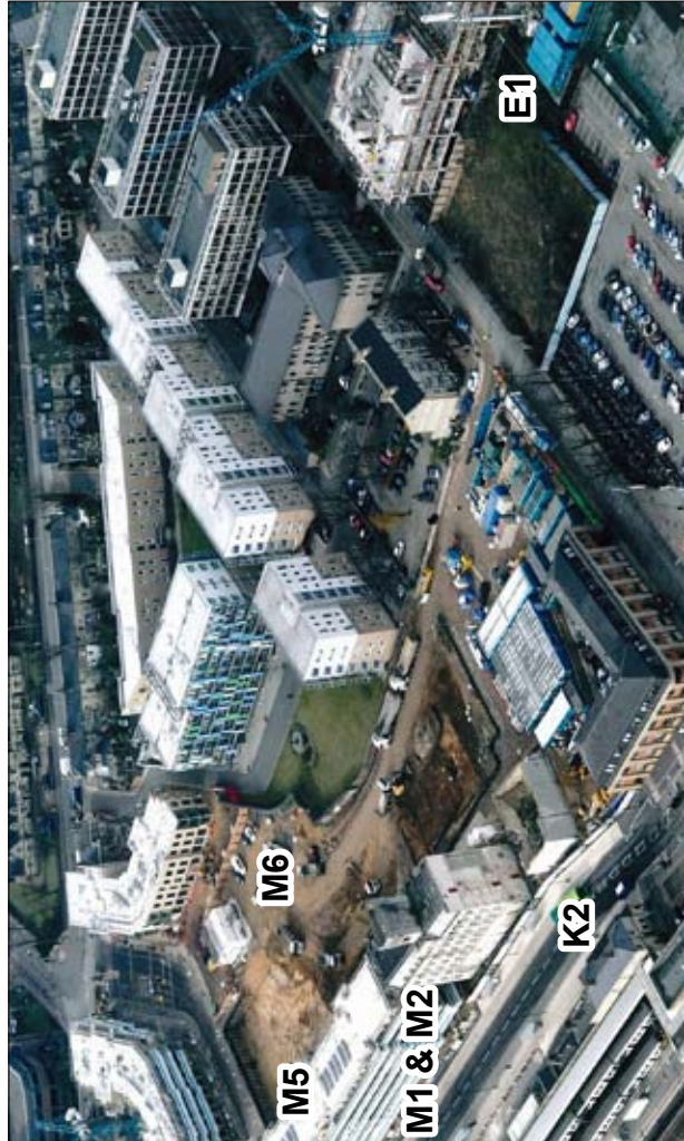
View looking south west showing buildings M1 & M2, M5, M6 and K2 (Fosters Mill to be converted) and E1.
