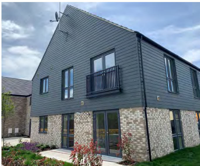
Buildings should aim to keep simple lines to the façades, with efficient building envelopes. Anstey Way, Trumpington, Cambridge. Rock Townsend
