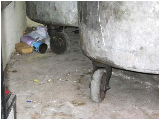
Rotting Food and litter on the chamber floor, under the bin.
