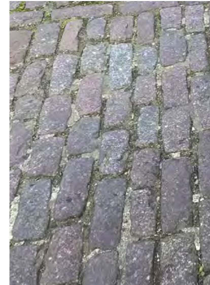
Staggered bond (rectangular setts)
