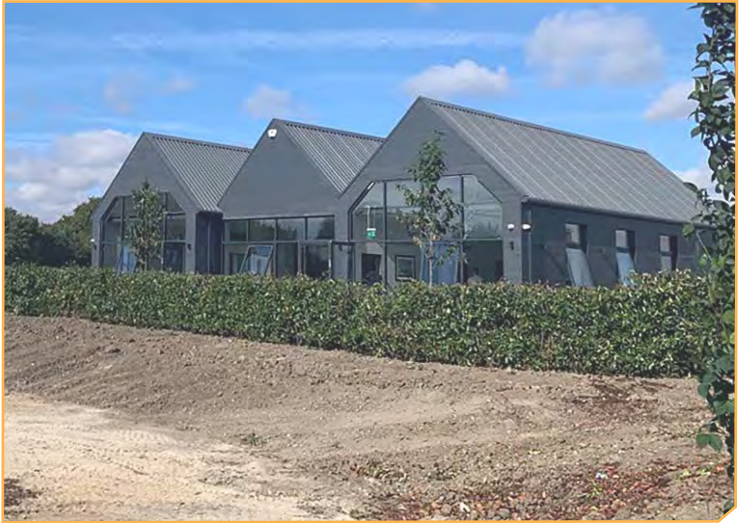
Site Office Temporary Building
