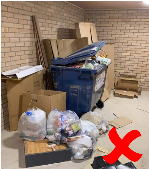
Fig 12 Bad bin store design – too much space in store allowing fly-tipping of cardboard
