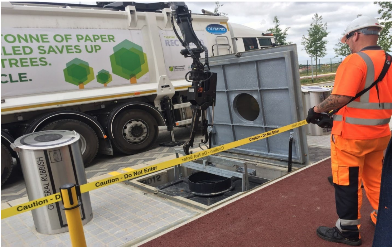
Fig 19 Underground bins hook-lift system in the ground
