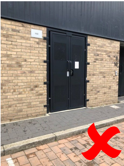
Fig 7 No drop kerb & pavement too narrow for 1100 litre bins
