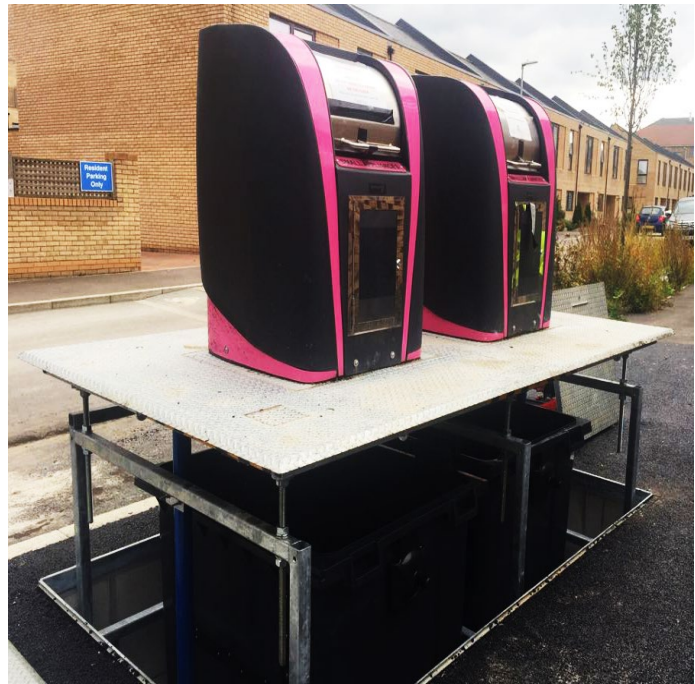
Fig 17 Double Hydraulic bring banks collecting small electrical appliances
