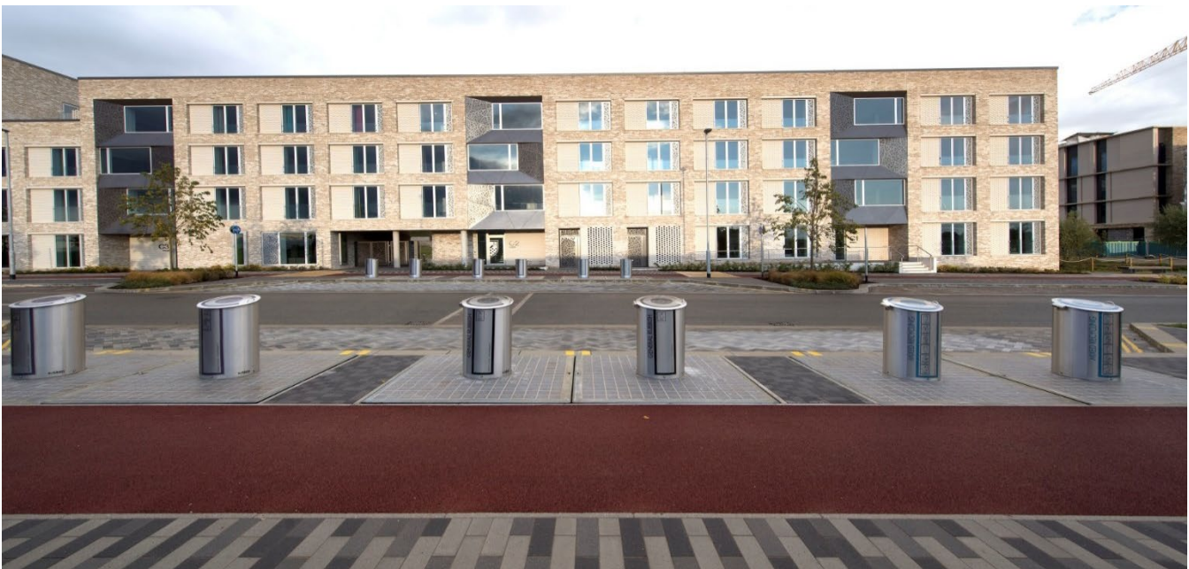
Fig 18 Underground bins hook-lift system streetscape
