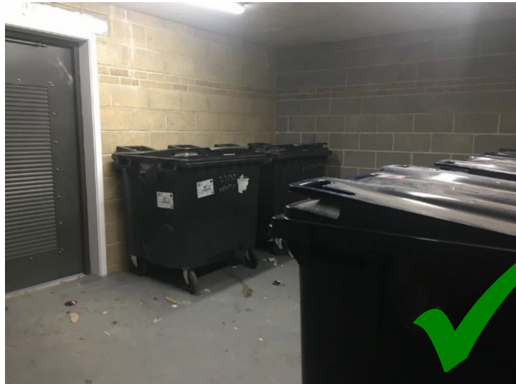
Fig 13 Good bin store design – bins fit in the bin store without too much excess space
