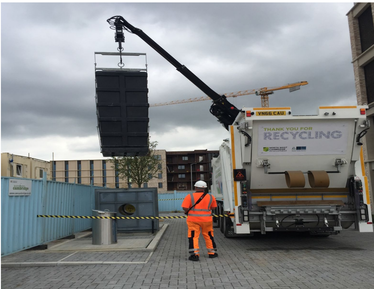
Fig 20 Underground bin hook-lift system out of the ground showing 5m3 container
