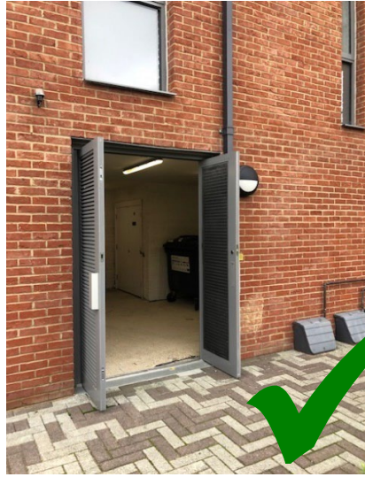
Fig 6 Double doors – stay open while collection takes place, with door bolts, hooks or automatic opening systems
