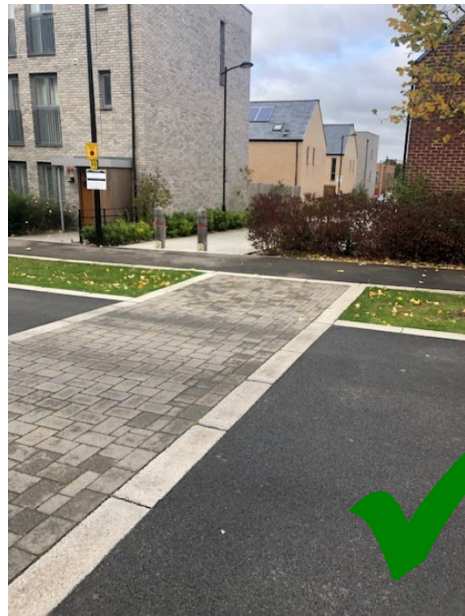
Fig 11 Swales is slabbed to allow 1100 litre bins to be easily moved to the roadside for collection
