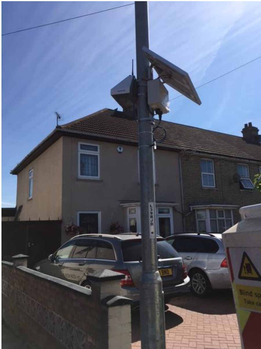
Figure A8 Monitor 292 Coldhams Lane
