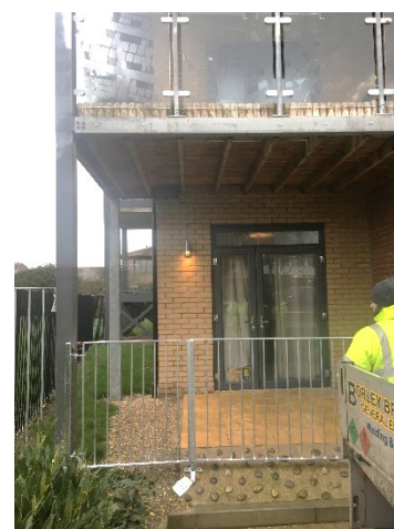
New balcony fencing and enclosure at Upperhall
