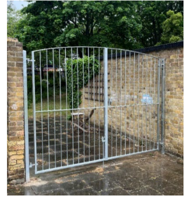
New security gating at Staffordshire
