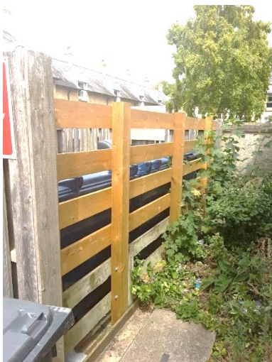
Example of a quick, small fencing repair, rapidly commissioned and completed
