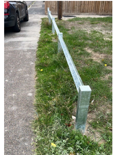
Very different galvanised fencing style at St Thomas Square, to prevent parking on the grass verge, with new bulb planting beneath it
