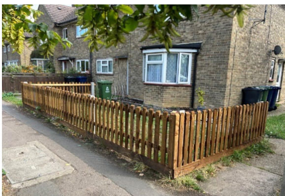
New wooden estate fencing at Whitehill
