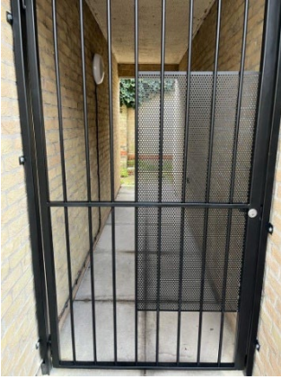
One of a pair of similar new security gates at Ditchburn Place sheltered scheme, Which cost £595 each
