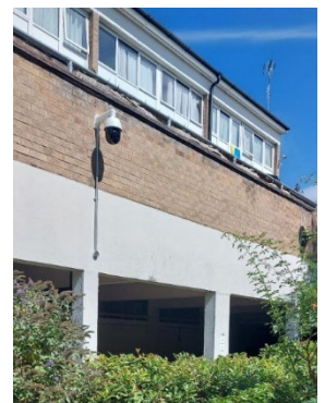
New CCTV installation at Bermuda
